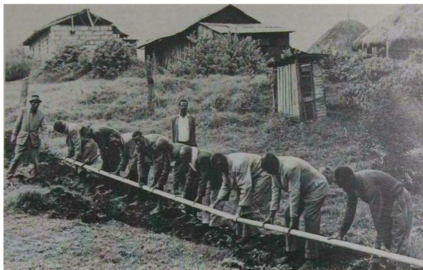
A water pipeline is laid by villagers in a self help effort near Nairobi. Curricula and training programmes have been developed in rural regions to maintain water supplies and sanitation facilities.
