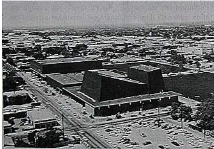
The new Community and Convention Center in Fresno, California. The three-building complex made from Cor-TEN, a special highstrength low-alloy steel developed by United States Street was designed by Robert Stevens Associates Fresno, Calif., and Adrian Wilson & Associates Los Angeles, Calif.
