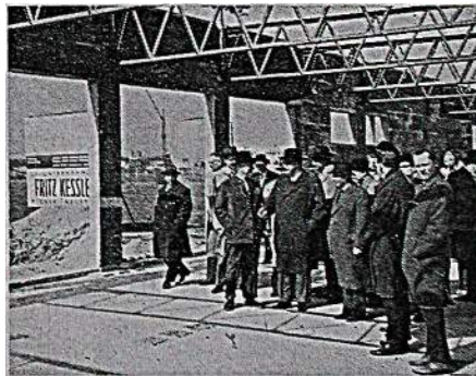
The Austrian Federal Chancellor Mr. Julius Raab visiting the laboratory building, of the International Atomic Energy Agency at Seibersdorf near Vienna, to celebrate the completion of a stage of its construction
