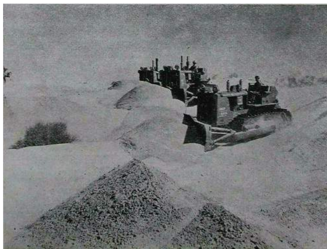
Preparations for laying the 24 inch oil pipeline Hassi-Messaoud Bougie. (Photo Grep).
