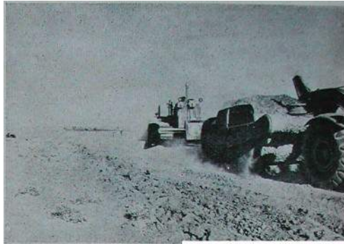
Aerodrome under construction in Afghanistan
